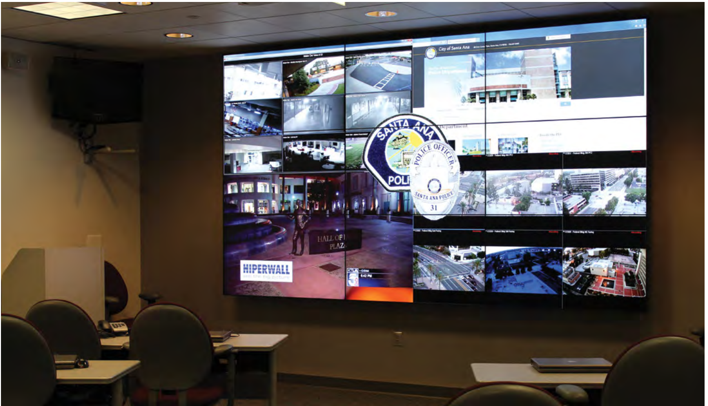
Hiperwall visual command center at the Santa Ana Police Department in Southern California.
